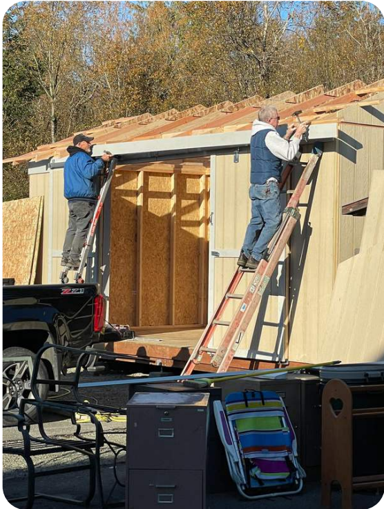
Construction of the furniture barn
